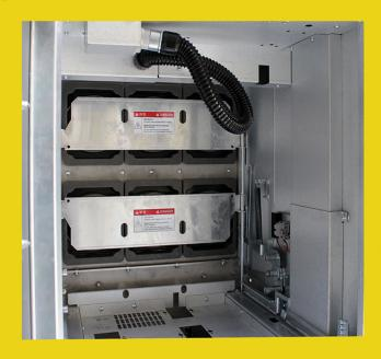
position of the vacuum circuit breaker to be clearly seen within the compartment. Besides, the position is also shown on the mimic diagram as well as optionally on the protection relay in case of customer request.
